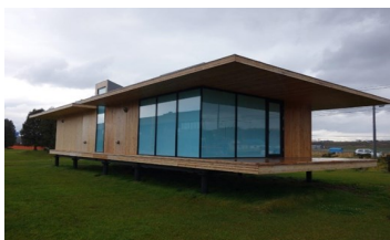
Fig. 1 Outlook of CLT Building
